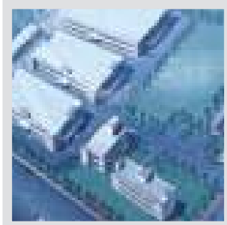
Wuxi Plant (China)
