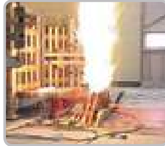
Short-Circuit Test / ACB Breaker Test
